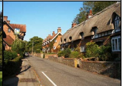
Crawley –thatch and timber frame and brick infill buildings. 1½ storey.
