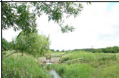
Itchen Valley Country park; sluice as part of restored water meadows.
